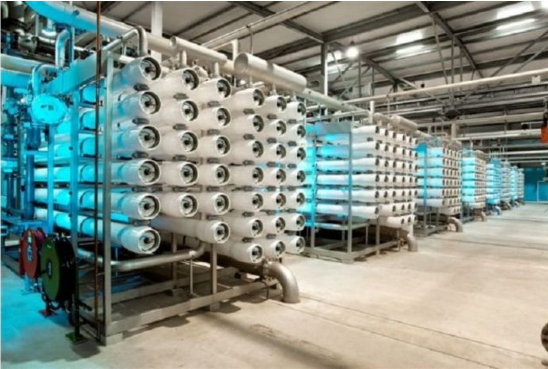
RO-installatie van Evides in de demiwater plant in de Botlek (foto: Evides).
